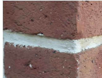
Efflorescences
